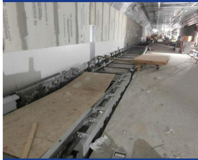
Beginning of wall tile installation inside the tunnel.
