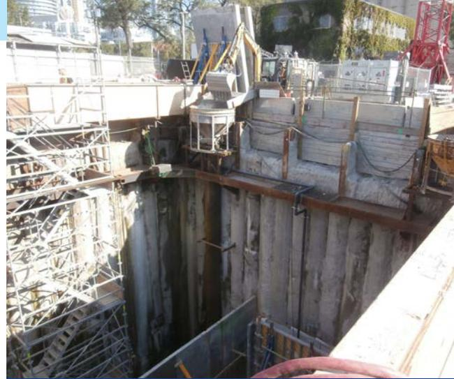
Backfill being placed into chute on mainland.
